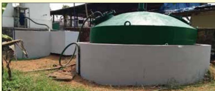
BARC model Biogas plant
