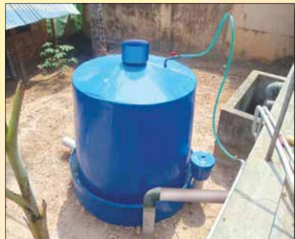
Figure 3.17 Portable Household Biogas Plant
