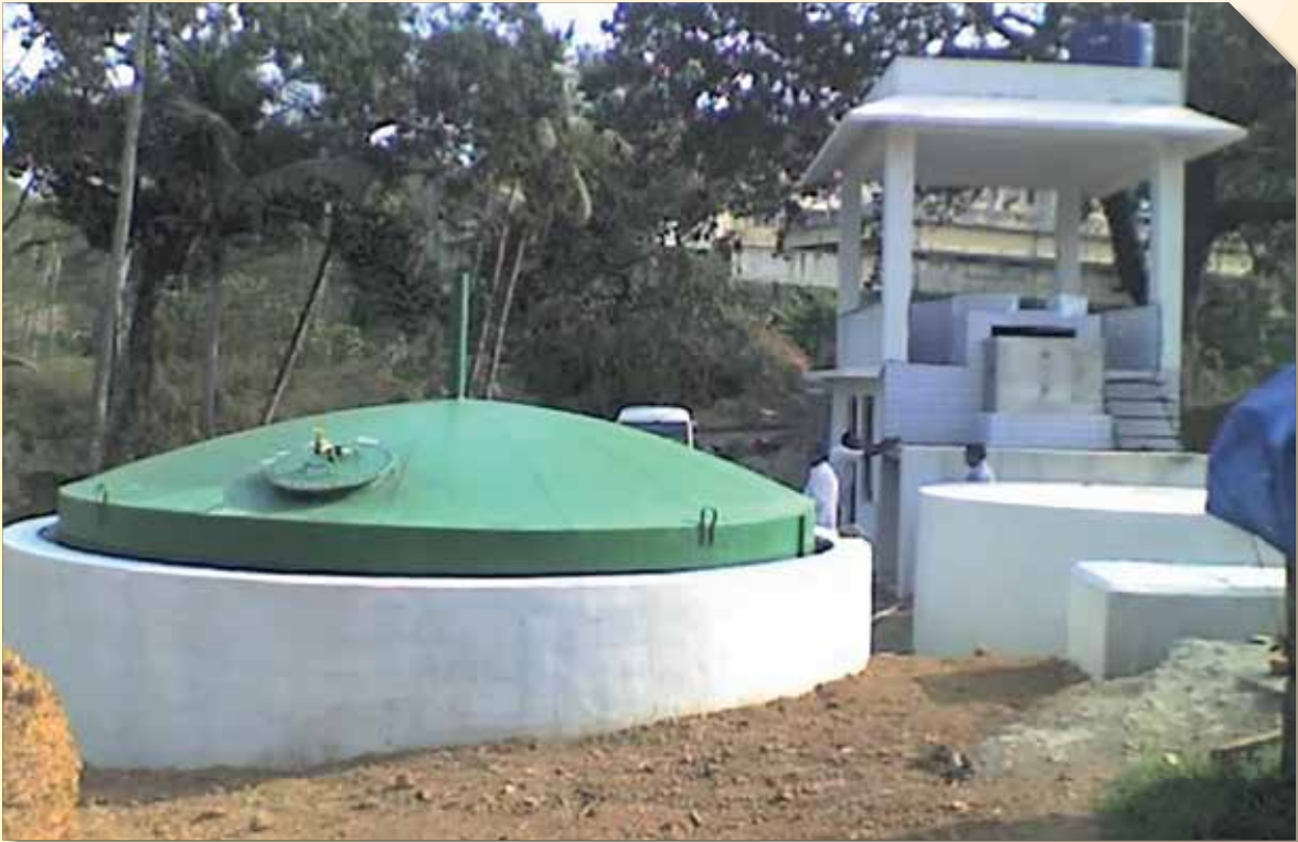
Bio Gas Plant
