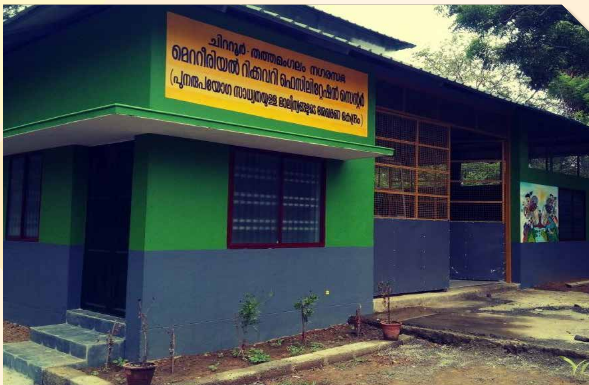
Material Recovery Facility (MRF) - Chittur Thattamangalam Municipality
